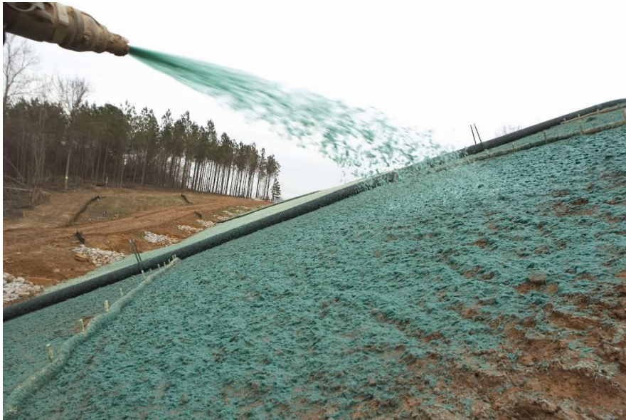
Hydraulically applied seed, mulch and binder
