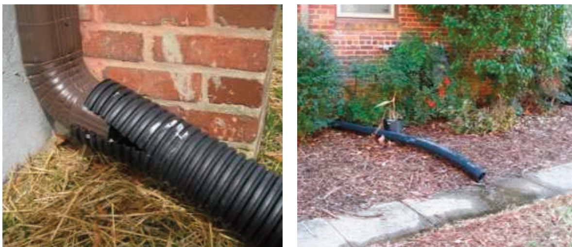
Figure 4: Poorly designed and installed downspout disconnections (Source: Carmen, NCSU).
