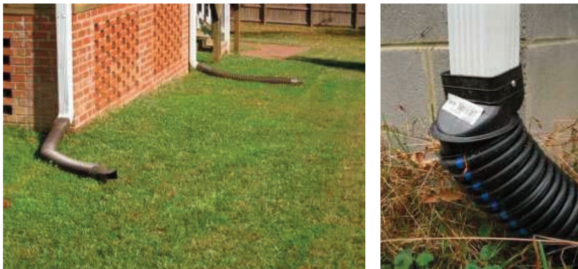
Figure 3: Disconnected downspouts on the left and a converter joint on the right (Source: Carmen, NCSU).
