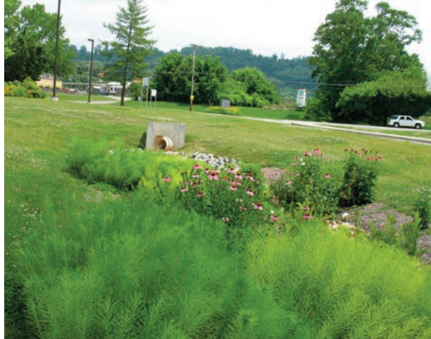
Figure 1: Bioretention capture water from parking lot in Powell, TN (Source: The SMART Center).
