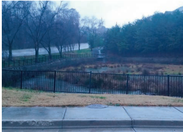
Figure 1: Wet pond with permanent pool storage and temporary detention in a residential setting (Source: SMART Center).
