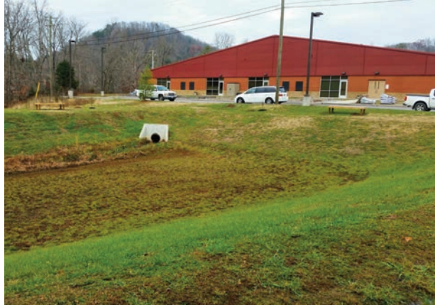
Figure 1: A dry detention basin with a pilot channel.
