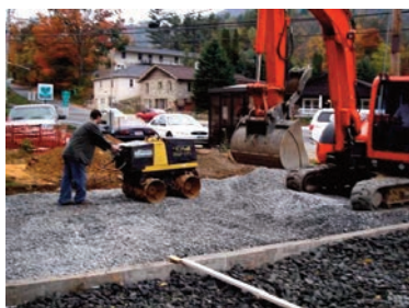
Figure 23: Compacting the open-graded aggregate base (Source: NCSU-BAE).
