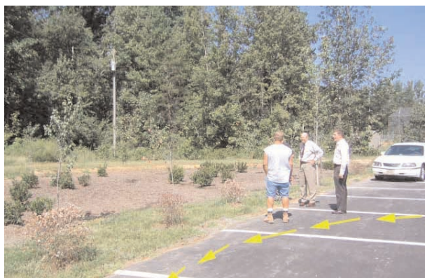
Some site runoff bypasses bioretention because of inadequate slope of filter strip.
