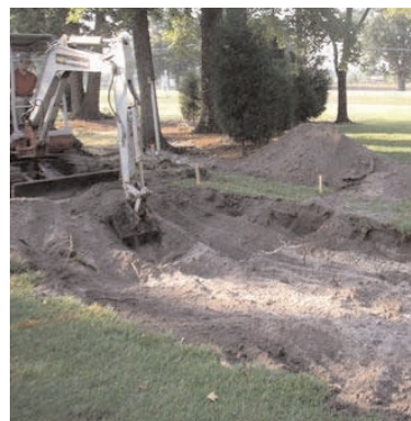
Figure 17: Where possible, excavate soil from the sides of the pavement area to minimize subgrade compaction from equipment (Source: NCSU-BAE).
