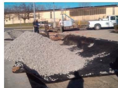
Figure 20: Filter fabric is installed on bottom and sides of reservoir layer (Source R.K.).
