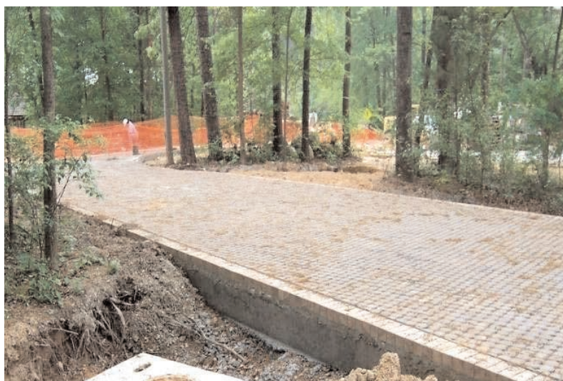
Figure 11: Edge restraint (Source: NCDENR).
