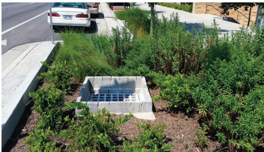
Figure 5.11: A drop inlet structure with a perforated riser as the outlet to a bioretention cell in Nashville, TN.
