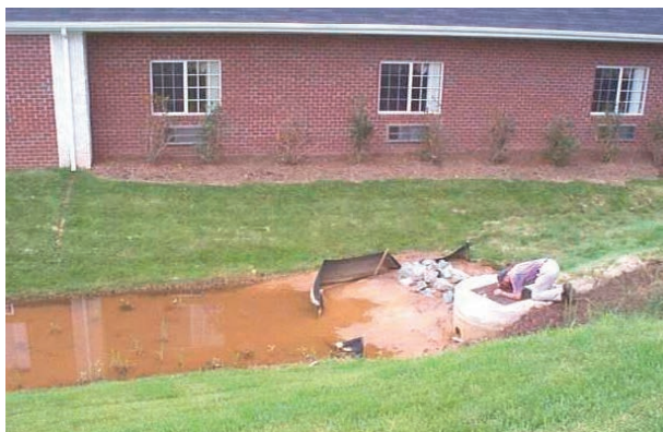
Bioretention area does not drain because of improper soil media, soils compacted during installation, and/or filter fabric under media.
