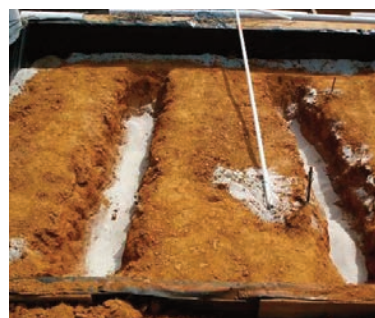
Figure 19: Trenching used to increase the soil infiltration rate (Source: Tyner).
