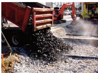
Figure 22: A dump truck deposits aggregate directly into excavated area for spreading (Source: NCSU-BAE).
