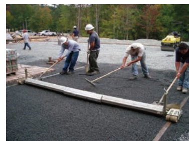
Figure 24: A 2 in. thick bedding course of aggregate is being screed smooth prior to placing the concrete pavers (Source: NCSU-BAE).
