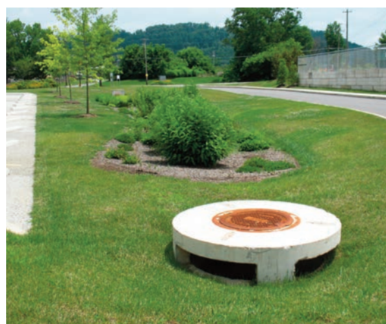
Figure 9: bioretention to capture runoff from a parking lot in Powell TN (Source: The SMART Center).
