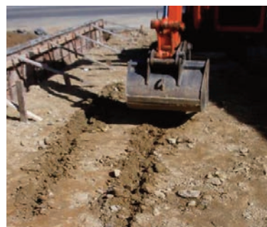
Figure 18: Ripping the soil subgrade increases its infiltration rate (Source: Tyner).
