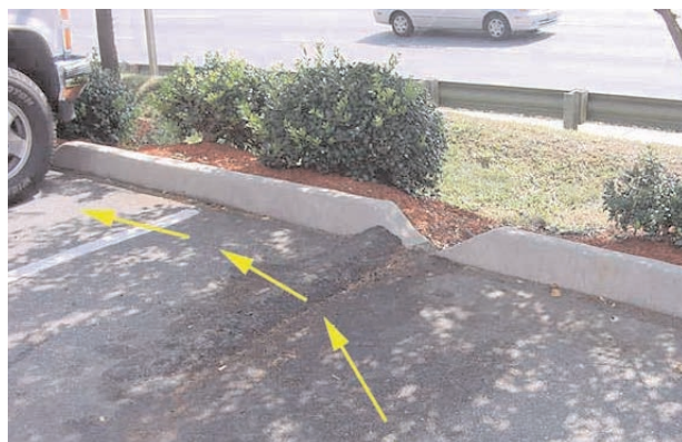
Site runoff bypasses bioretention swale because of small elevation changes during construction.
